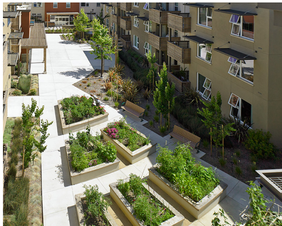
Fig. 4.8.6: Bioretention planters help manage site stormwater runoff as well as run-off from building roofs using downspouts.
