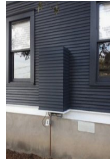
Figure 2.8.1: Example of a wall-mounted water heater enclosed in a cabinet.
