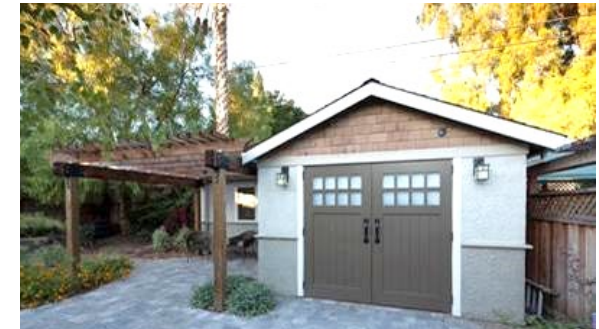
Figure 3.3.16: This ADU, created by the conversion of an existing detached garage, maintains the exterior appearance of a garage door and maintains the paved area in the driveway to the previous garage.
