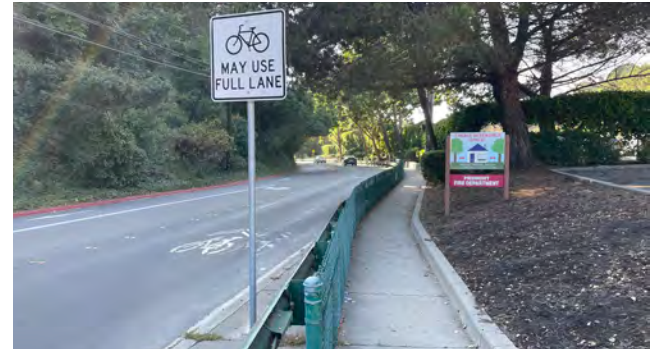
FIGURE 4.13: EXISTING CLASS III BIKE ROUTE, WESTBOUND MORAGA AVE
