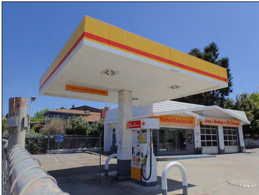
29 Wildwood Avenue. Northern (Grand Avenue side) fuel island and canopy. Office/service garage beyond. View east. LSA photograph 7/5/24.
