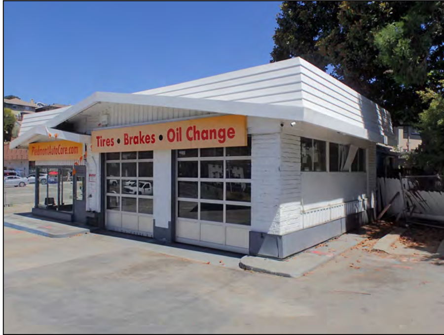
29 Wildwood Avenue. Office and service garage building. South façade and partial west façade. View northeast. LSA photograph 7/5/24.
