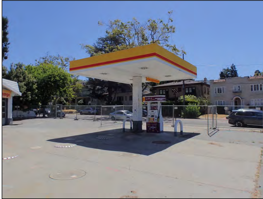
29 Wildwood Avenue. Southern (Wildwood Avenue side) fuel island and canopy. View southeast. LSA photograph 7/5/24.
