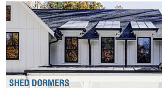
SHED DORMERS Shed dormers shall occur at a minimum of 50% of upper story openings.
