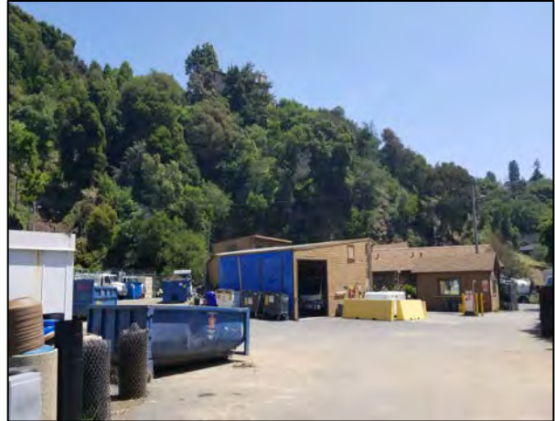
20. View of overhead power lines toward proposed tower location, East.
