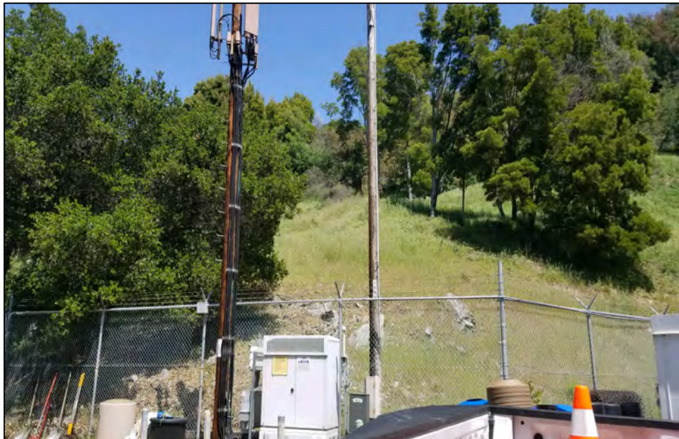
Figure 7. View to the north toward project location
