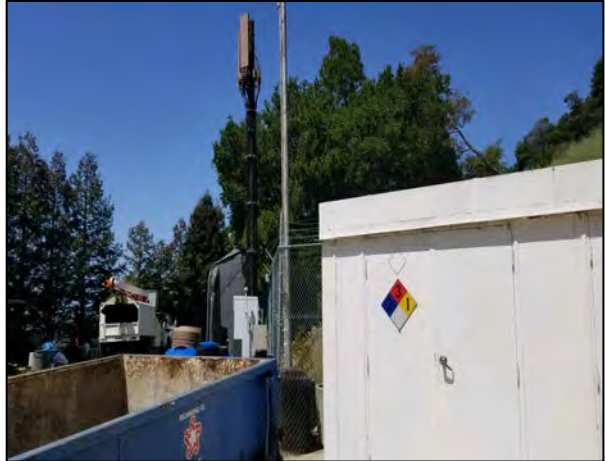
14. View toward proposed tower location, West.
