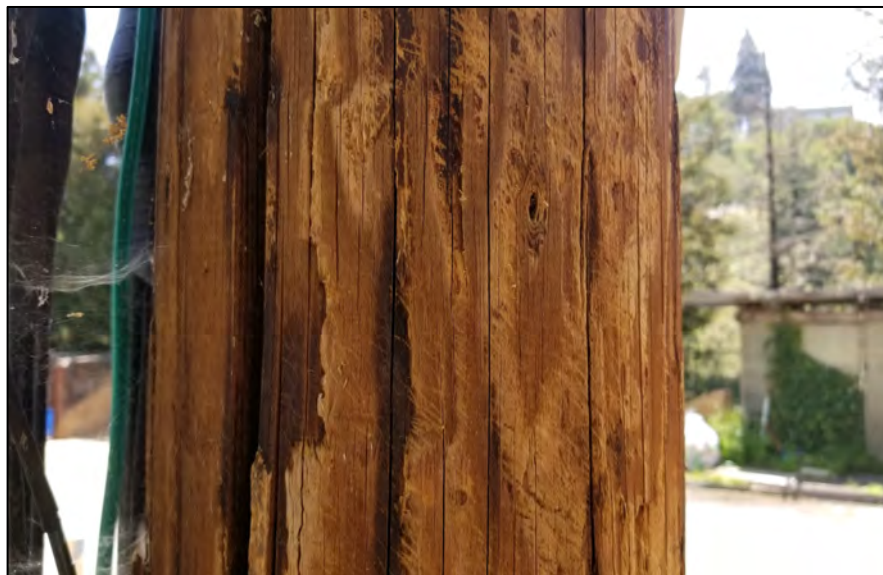
Figure 2. View to the south toward project location
