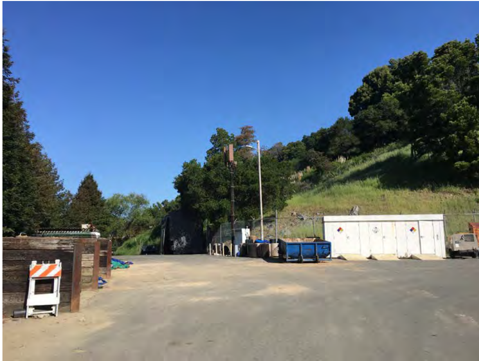
Site Photograph 1 – Looking northwest at Property and pole to be removed
