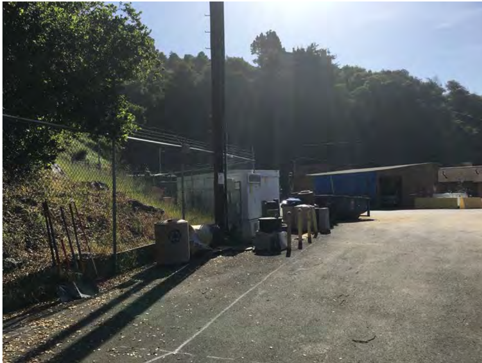
Site Photograph 4 – Looking east away from the Property and east at the tower to be removed
