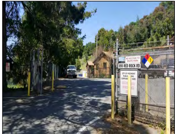
22. Overview of access entrance toward proposed tower location, Northwest.
