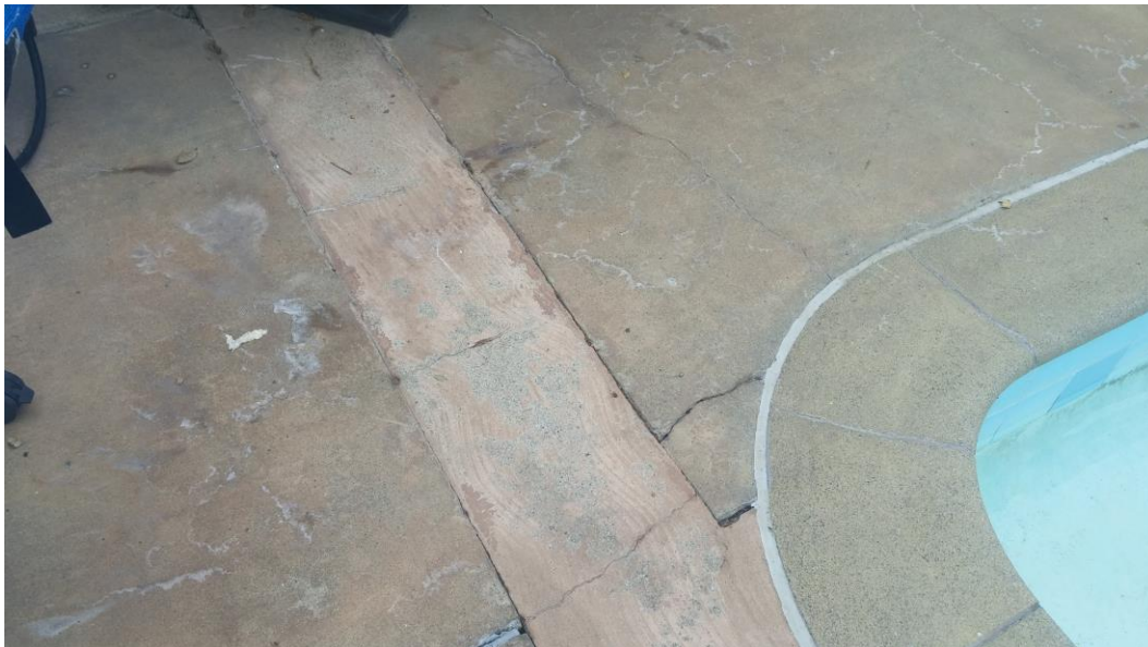
PP-2 Deck cracks, sections replaced
