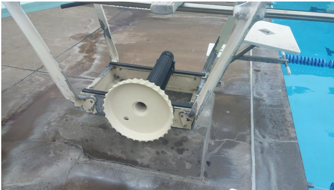
PP-16 Fulcrum not in the forward and locked position
