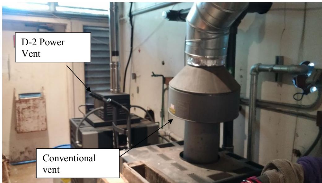
PP-40 Pool heater with standard flue
