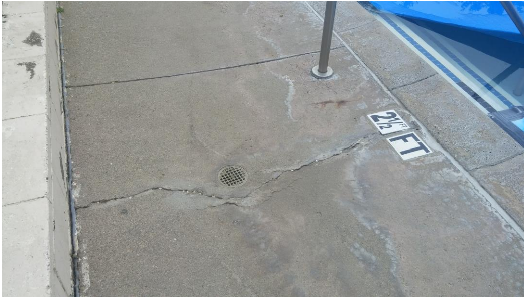
PP-1 Deck cracks, staining
