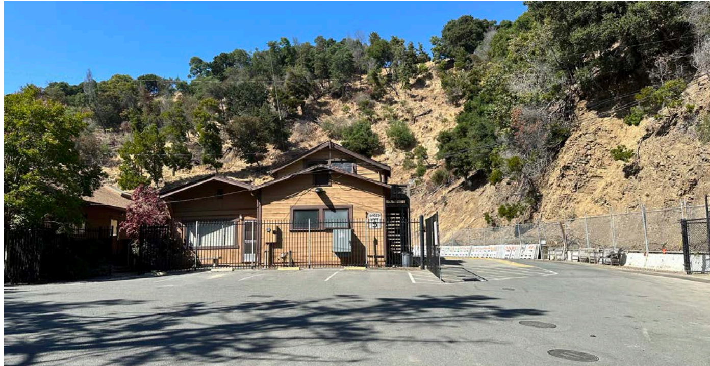
EXISTING CORP YARD OFFICE
